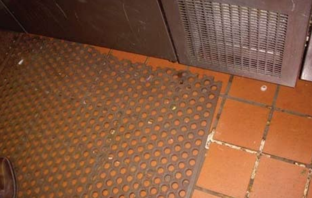
Left: Commercial hotel kitchen quarry tile after nine months of exposure to trans fats (oleic acid), followed by exposure to enzymatic cleaning agents. The grout used was 100% solids epoxy.
